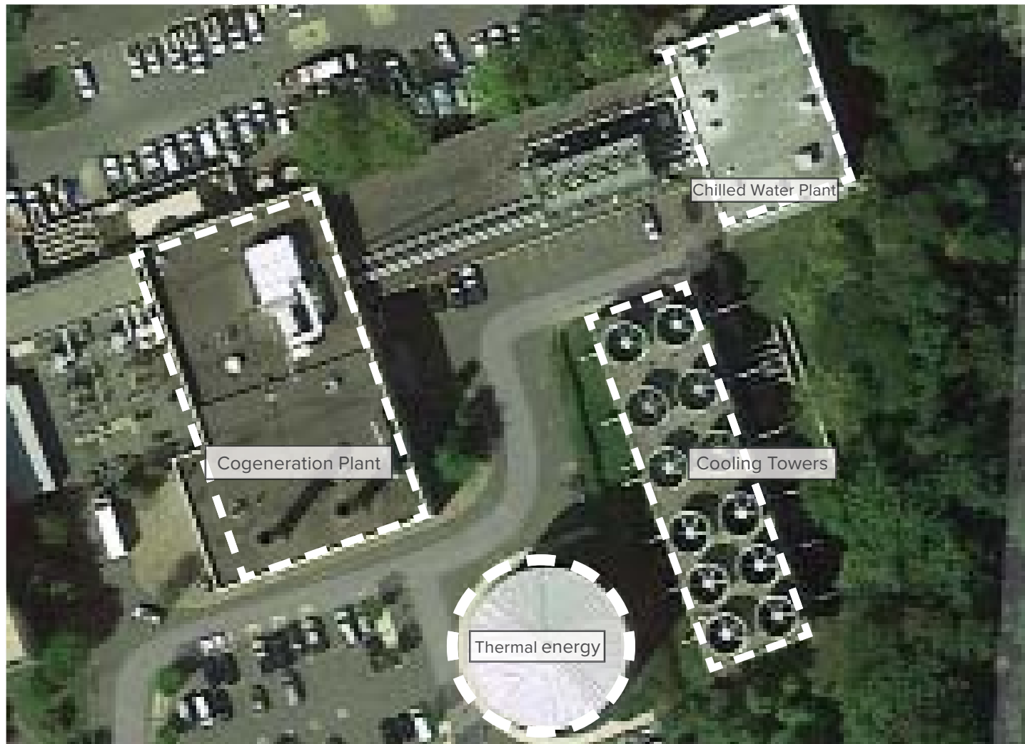
Figure 2. Princeton Co-generation Plant
