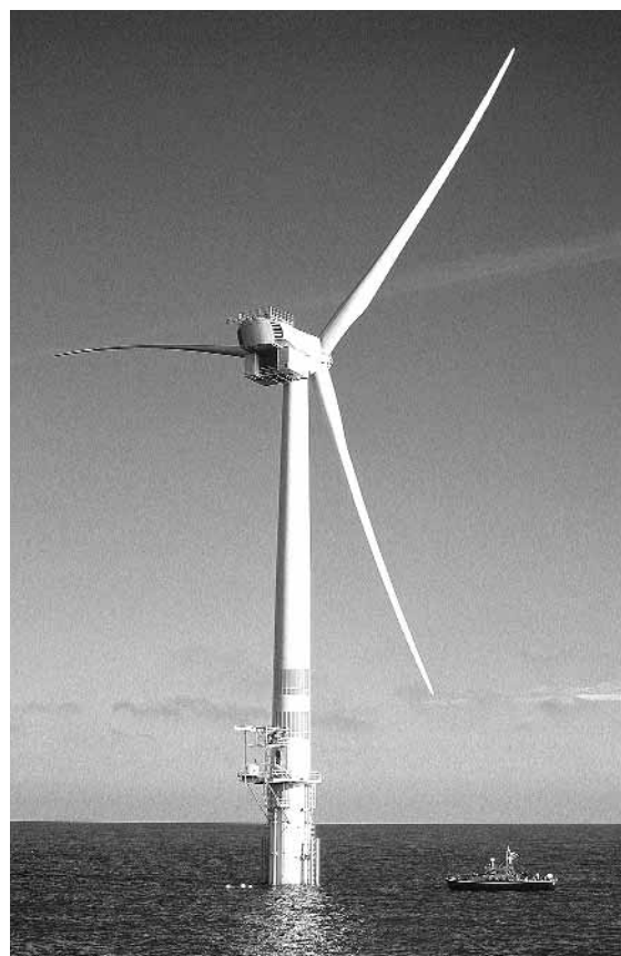
Arklow Bank Offshore Wind Power Facility, Ireland
